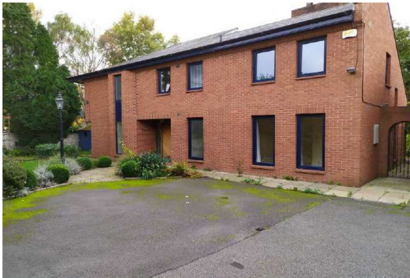
Plate 11 Elsinore, 97A Highfield Park, facing southeast
